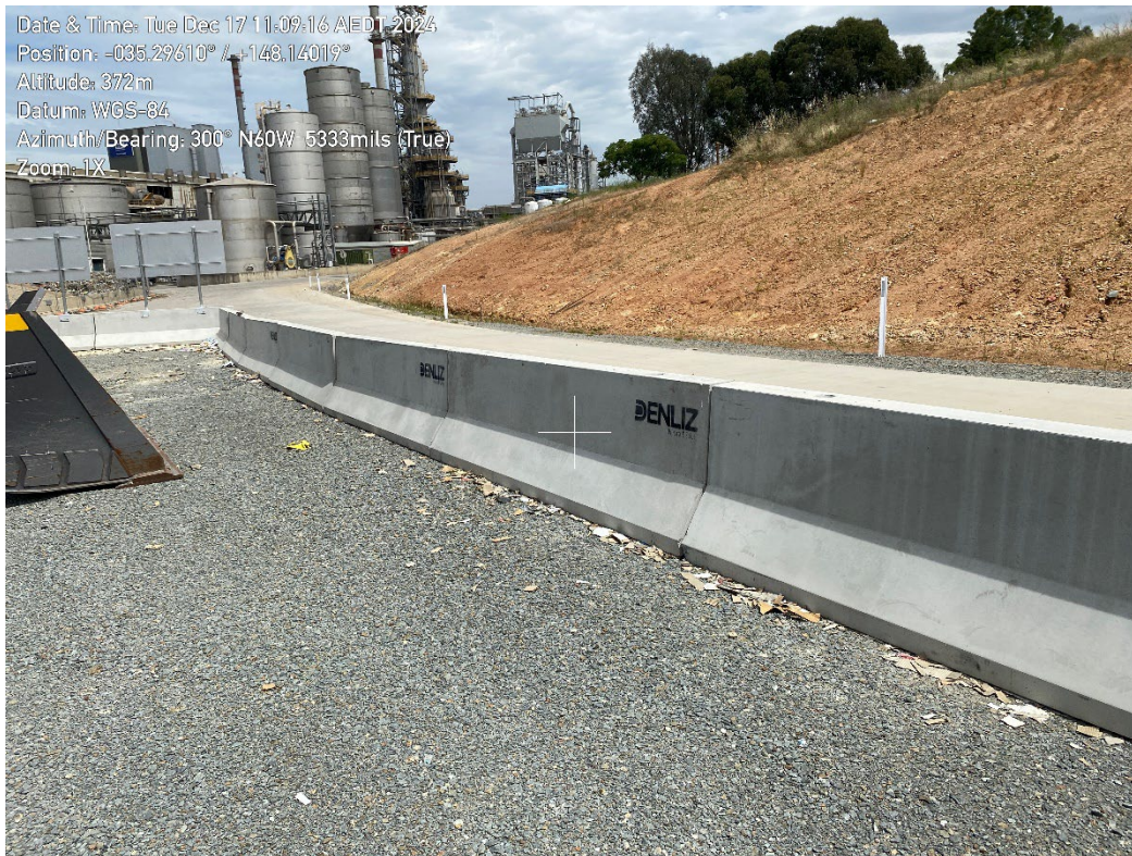
Photo 5 – New loop road with concrete partition to capture litter from waste storage area.
