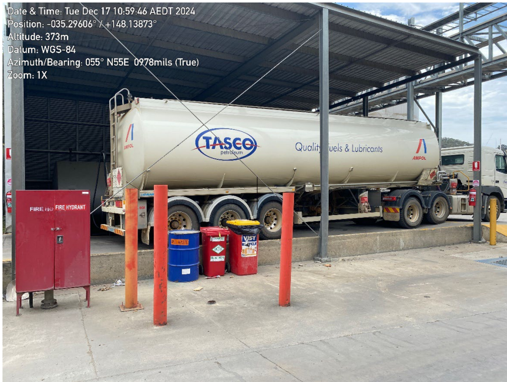
Photo 3 – Refuelling area with recycling bin, spill kit and spill waste disposal bin.
