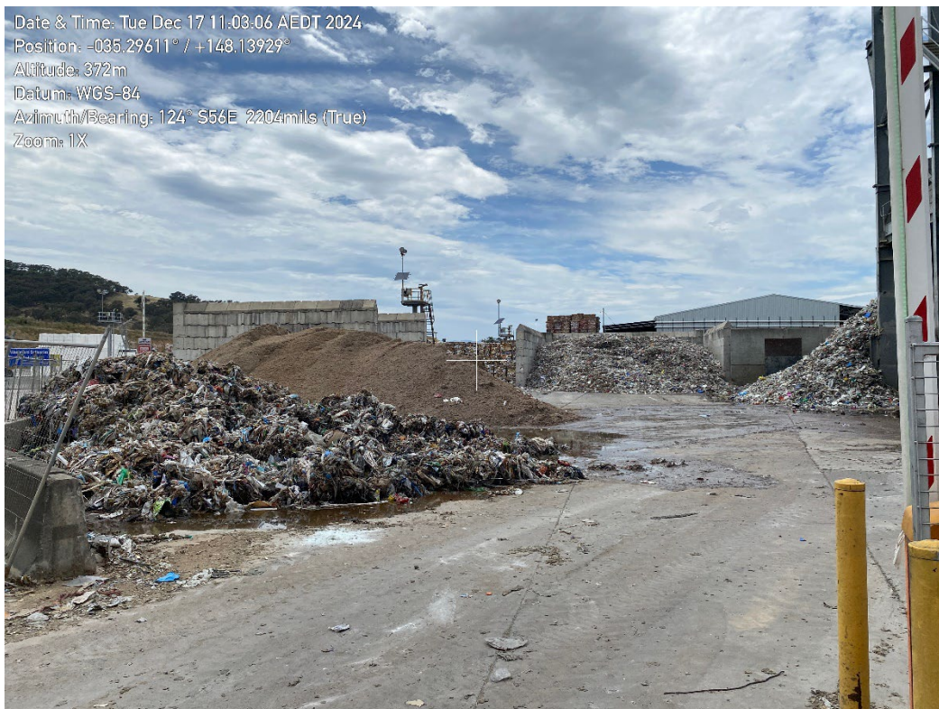
Photo 8 – Waste material stockpile to be reused (brown) and plastics and other wastes from paper recycling to be landfilled (foreground).
