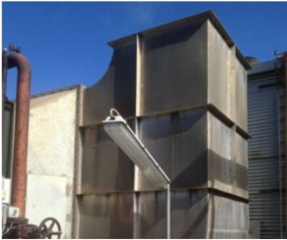
Vacuum Pump 9 (Paper Machine Hood Vent Exhaust)
