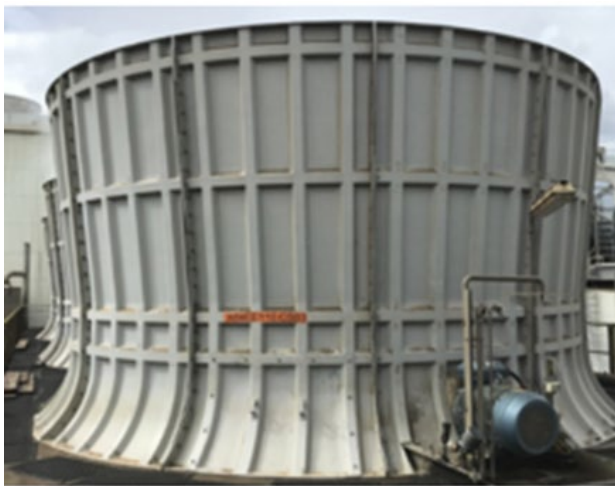
Cooling Tower (#1 Paper Machine Side)
