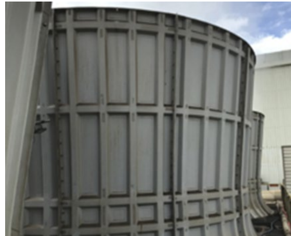
Image 6. Cooling Tower (#2 Paper Machine Side)
