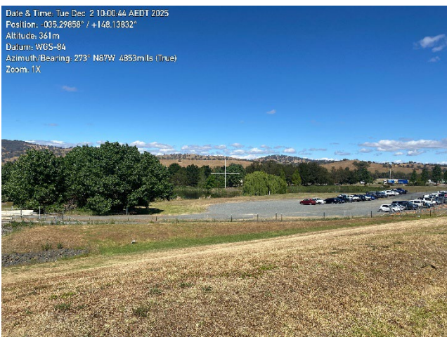
Photo 9 – Lined and vegetated stormwater channel (left), stormwater ponds (centre).
