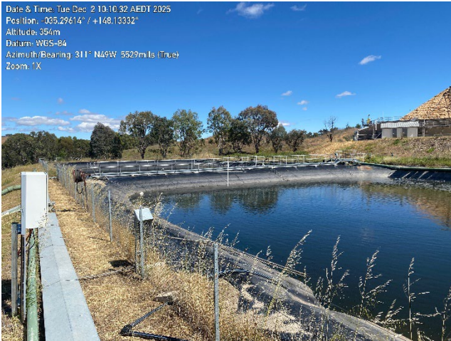
Photo 11 – Cooling pond water is treated and reused for either irrigation or transferred back into the plant and reused as Cooling Tower make-up water.
