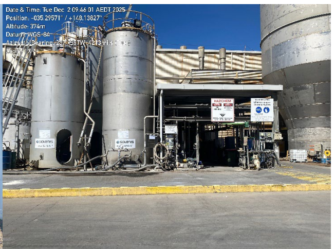
Photo 4 – Bunding of hazardous materials area.
