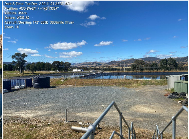
Photo 12 – 6 megalitre dam only used during mill shutdown. Water is reused in mill untreated.
