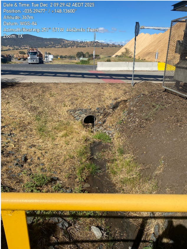
Photo 13 – Runoff captured and directed to WWTP.
