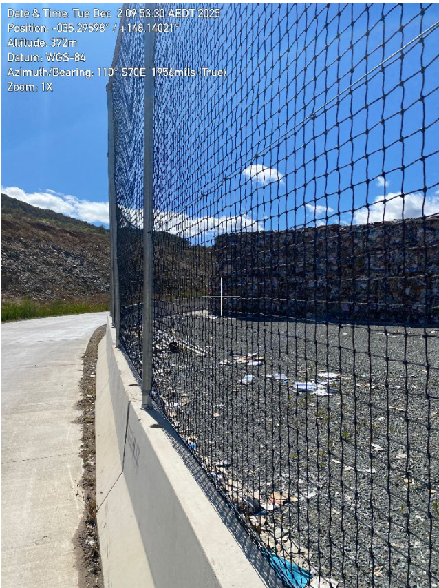
Photo 21 – Waste storage area netting and loop road.
