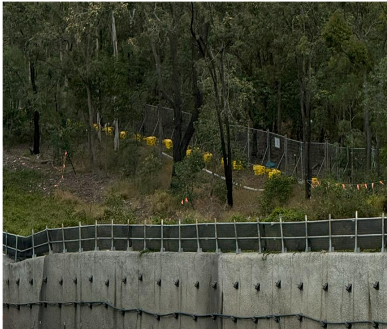
Photo ID: 9 – Fencing observed surrounding the Development Area at the Site.
