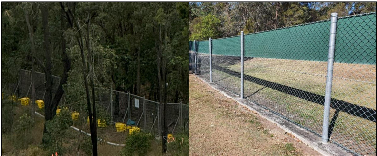
Figure 6 Temporary fencing at the Site (left) and koala exclusion fencing example (right)
