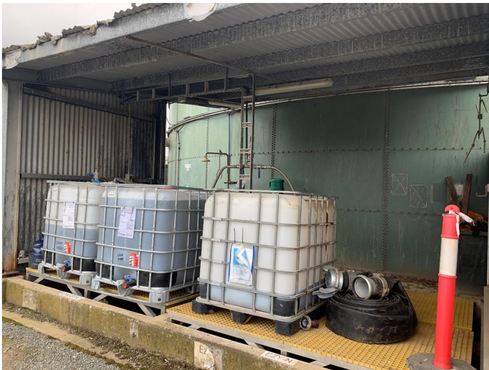
IBC chemical storage in appropriately bunded and covered area
